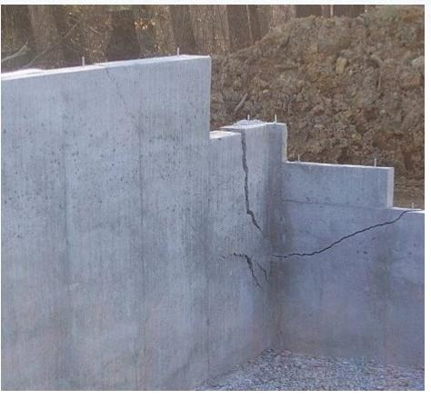
Cold-weather damage to a concrete foundation (Photo courtesy of InspectAPedia®, http://inspectapedia.com/index.php).
